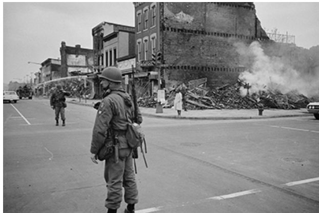
FIGURE 29.17 Many businesses, such as those in this neighborhood at the intersection of 7th and N Streets in NW, Washington, DC, were destroyed in riots that followed the assassination of Martin Luther King, Jr.
